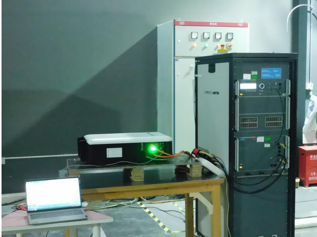
Photograph 7: Set-up for Surge
